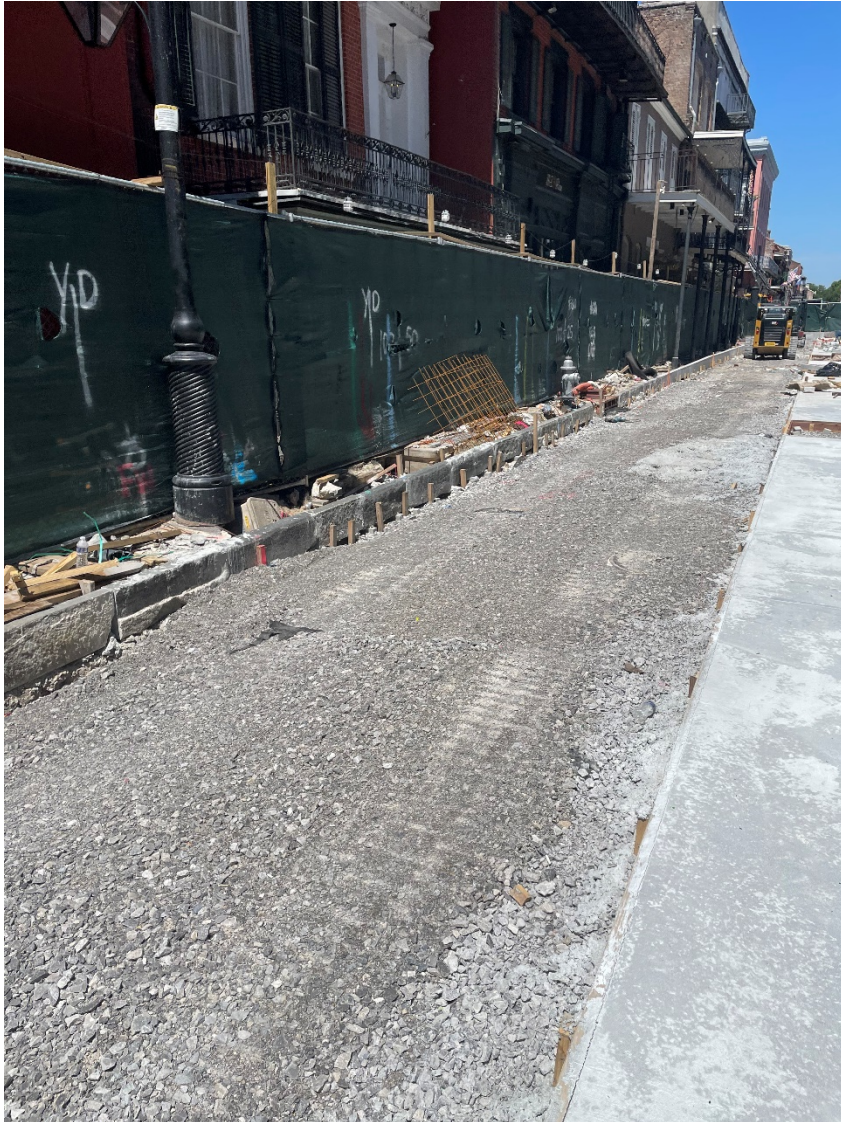
Photos: progress on the 600 block of St Peter St
